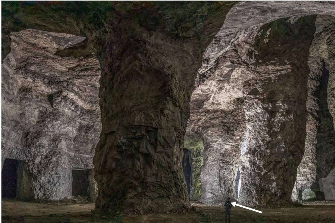
Long-term stability for underground excavations
